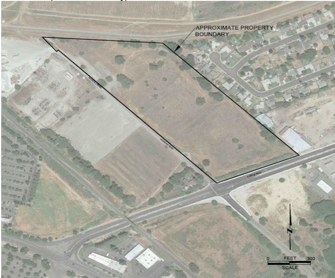
Aerial View of the subject 19.2-acre parcel at 6035 Avondale Ave., Linda, CA., future home of the Yuba- Sutter NextGen Transit Facility.
