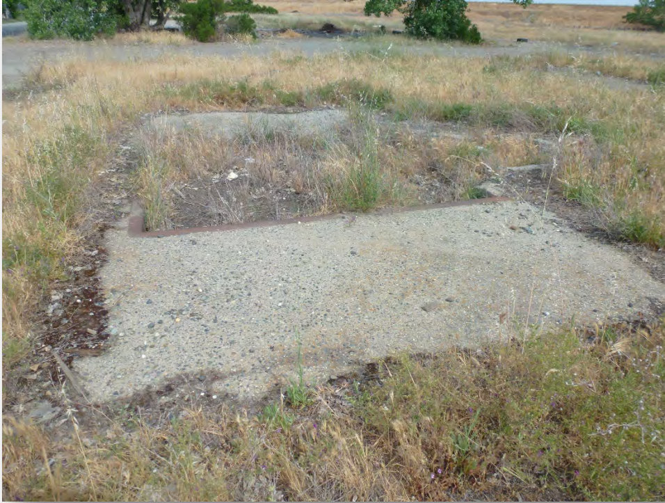
Photo 11. Slab with sump, northwestern property boundary.
